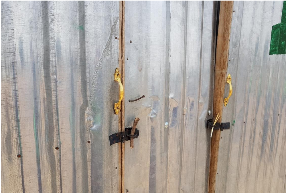
Latrines have basic external locks to prevent the doors flapping open in the wind. Photo: Marion O'Reilly/Oxfam
