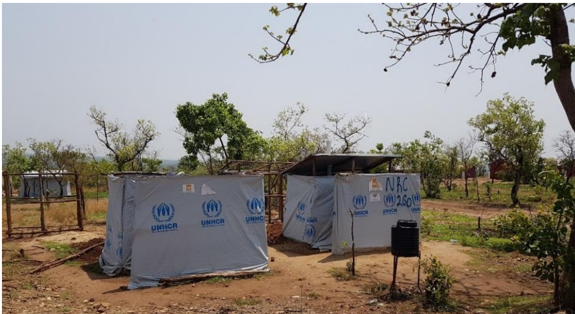
A new bathing shelter (left), latrine (right) and handwashing stand
